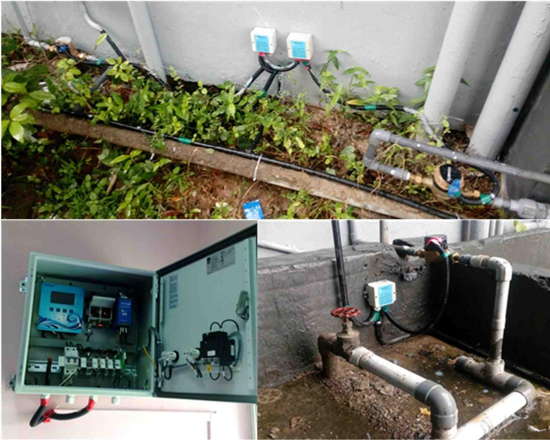
Fig.4. Sub metering using AMR Water metering system
