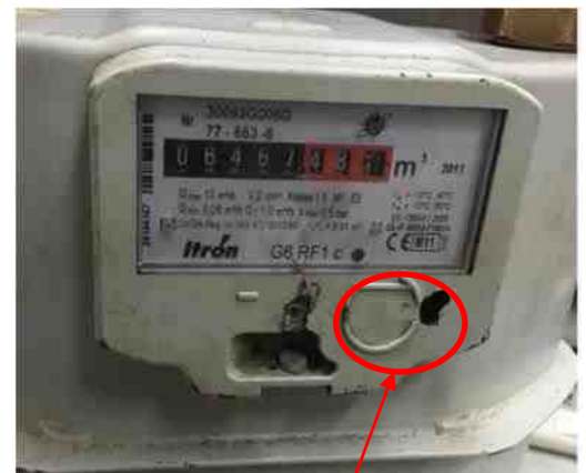
Fig 2- Meter tampered (Blocking of transfer gear assembly)
