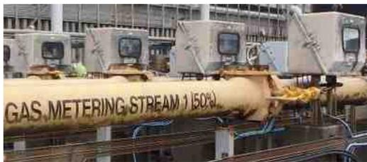
Fig 2. Gas Custody Transfer Orifice Meter
