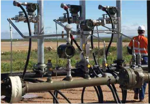
Fig 32. Orifice Meter with Prognosis on a Plunger Lift Well.
