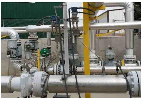
Fig 11. CEESI 8" Orifice Meter Wet Gas Test.
